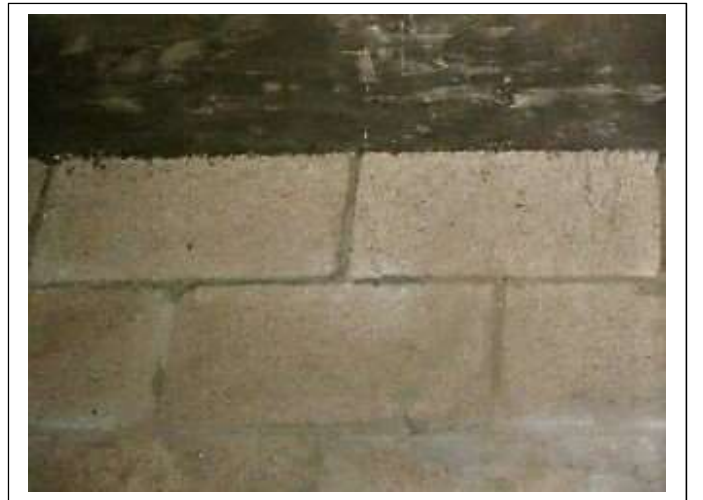
REINFORCED CONCRETE WALLS
