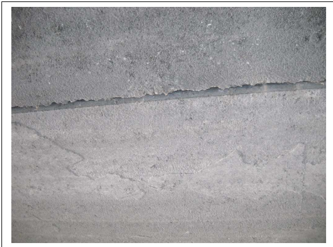
REINFORCED CONCRETE ROOF DECK
