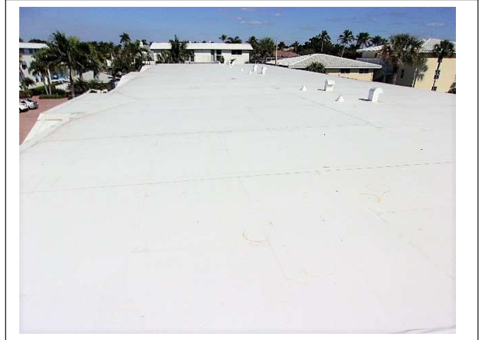
ROOF COVERING SYSTEM – The roof covering system is fully functional with no observable deficiencies.
